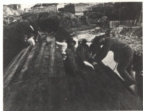
DRIVING A STAVE — Millwright Donald Gauthier springs the staves apart as other construction workers slide the final one between its tongue and grooved neighbors, and drive it into position against the butt plate. At the time this picture was taken, about 40' of penstock was still to be built before the job was finished.
