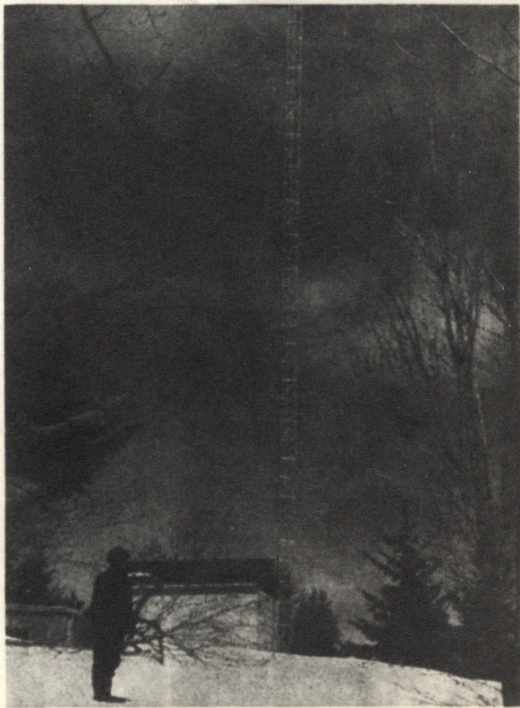
CATES HILL TOWER—Maurice Quinn, forest engineer in the Woods Department, stands at the base of the new radio tower on Cates Hill. Concrete block building holds transmitters and receivers, both those of State Forestry Department and Brown Company Woods Department. Only the lower half of the 120' high tower is shown in the above picture.
