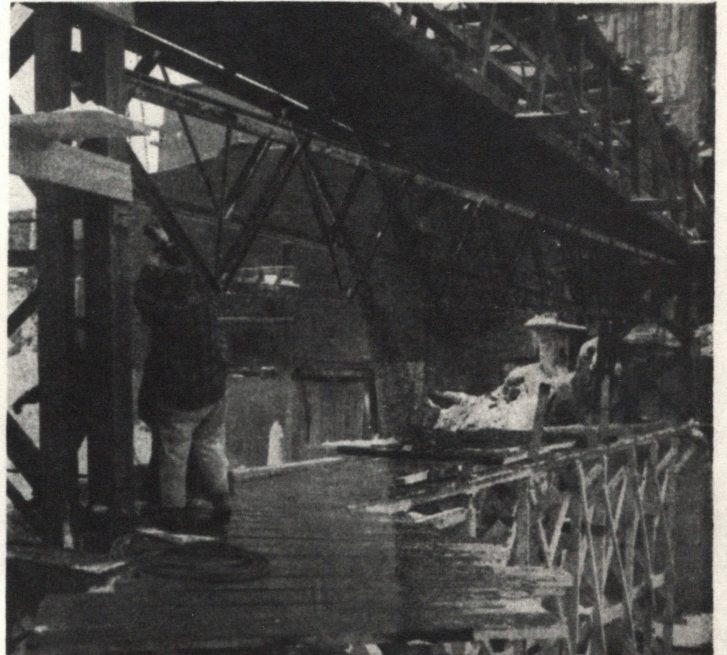
LIFTING TRUSS —Chain falls were used by construction crew to lift 80' long steel truss, weighing 4 tons, to point directly beneath wooden bridge.
